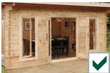
Slab base perfectly level across both the width and depth.
